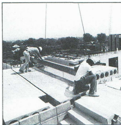
The floor system is installed...
